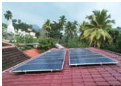
Providing 15 numbers of 340W Solar panels for Installation of 5-kW solar PV system at the Bible, kotagala Piyangala Purana Temple
