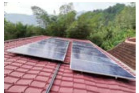
Providing 15 numbers of 340W Solar panels for Installation of 5-kW solar PV system at the Bible, kotagala Piyangala Purana Temple
